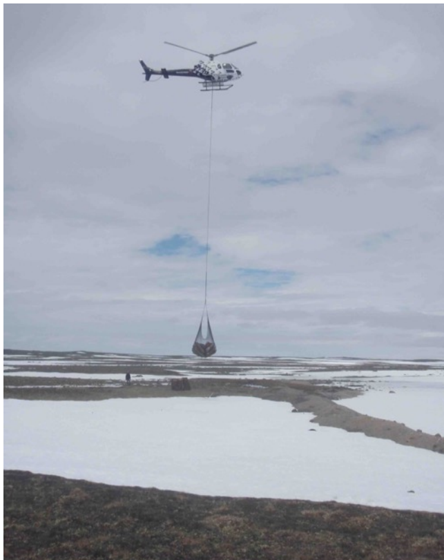
Figure 28 KG-2 during rehabilitation activities, June 2018
