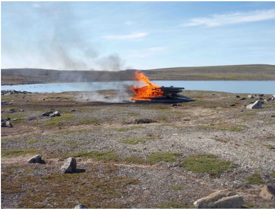
Figure 35 SW-27C during rehabilitation activities, July 2018
