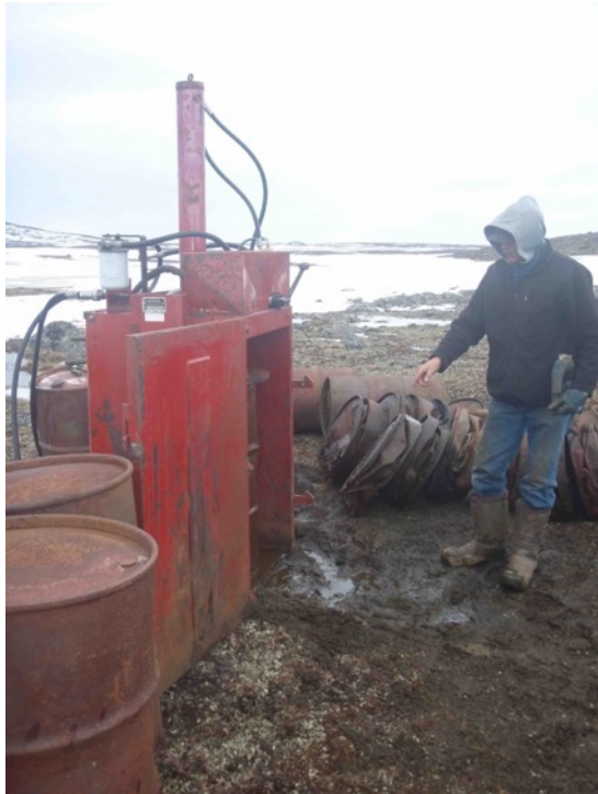
Figure 21 KG-1 during rehabilitation activities, June 2018
