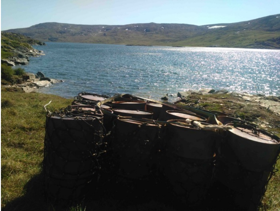
Figure 31 Watts Lake-2 during rehabilitation activities, July 2018
