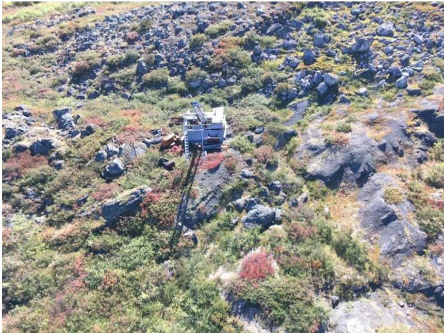
Figure 1 Jordon Lake-2 during inspections, September 2017
