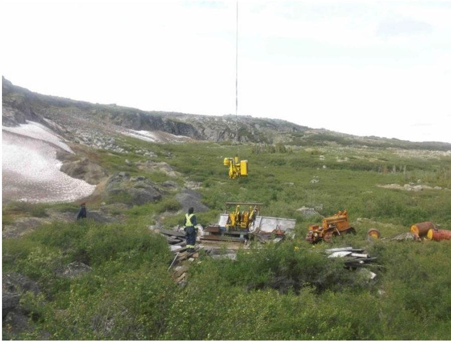
Figure 3 Jordon Lake-2 during rehabilitation activities, July 2019
