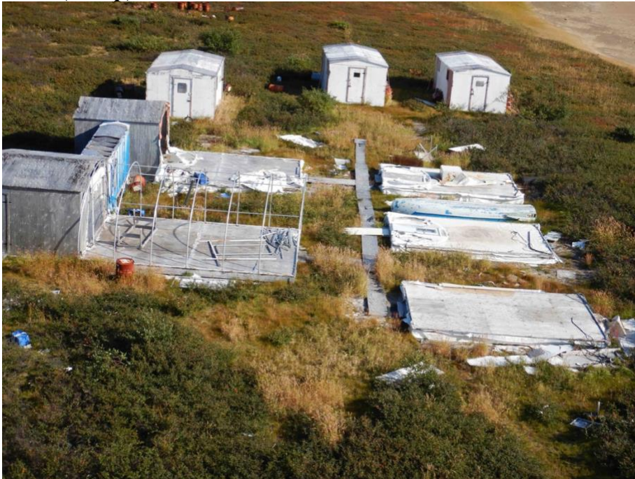
Figure 15 GR-3 Camp during inspections, September 2019
