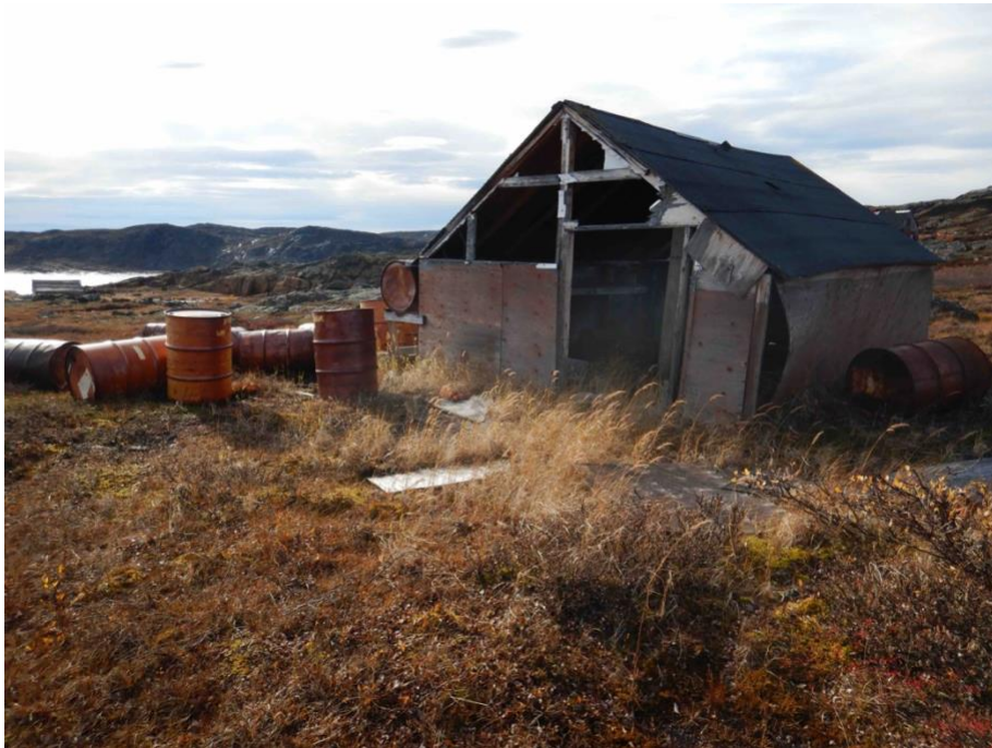
Figure 22 Weymouth camp during inspections, September 2019
