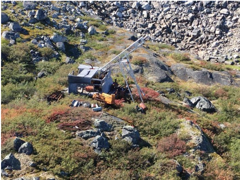
Figure 2 Jordon Lake-2 during inspections, September 2017
