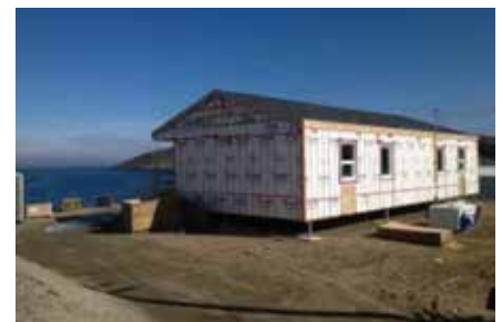
Figure 5: Housing construction in Nunavik
