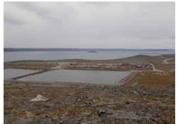
Figure 23: Wastewater lagoon in Kangirsuk with the northern landfill in the background
