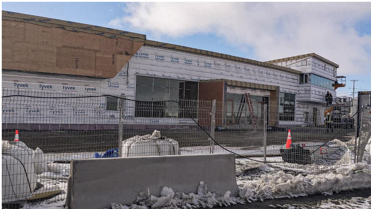
Construction of the airport terminal in Salluit will soon be completed.
