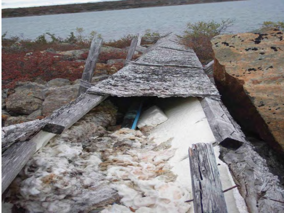
Photo 9 Wood covered pipeline found on site KAW-35
