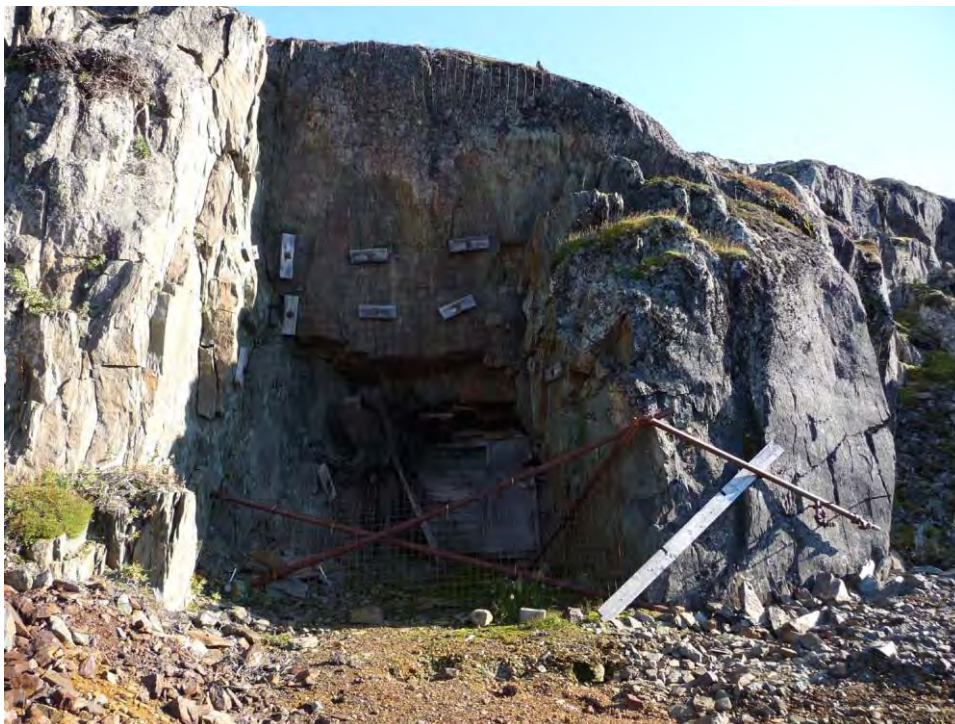
Photo 38 Sector 4: Opening leading to the gallery having been secured, PJ-1 site (September 16, 2011)
