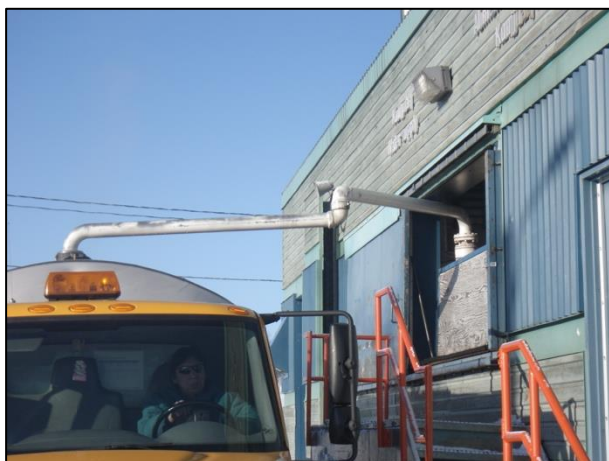
Photo 5. Filling of a water truck at the water treatment plant for distribution in the village (2014, KRG)
