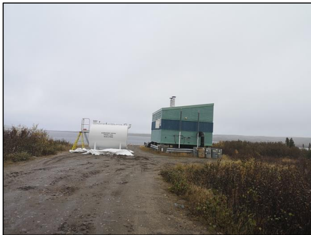
Photo 2. Pumping station on the shore of Lake Stewart (September 2019, KRG)
