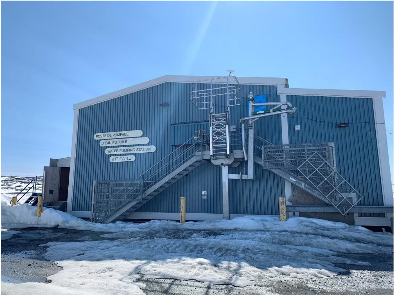
Figure 4. Exterior view of the drinking water treatment plant. Photo taken on May 19, 2024.
