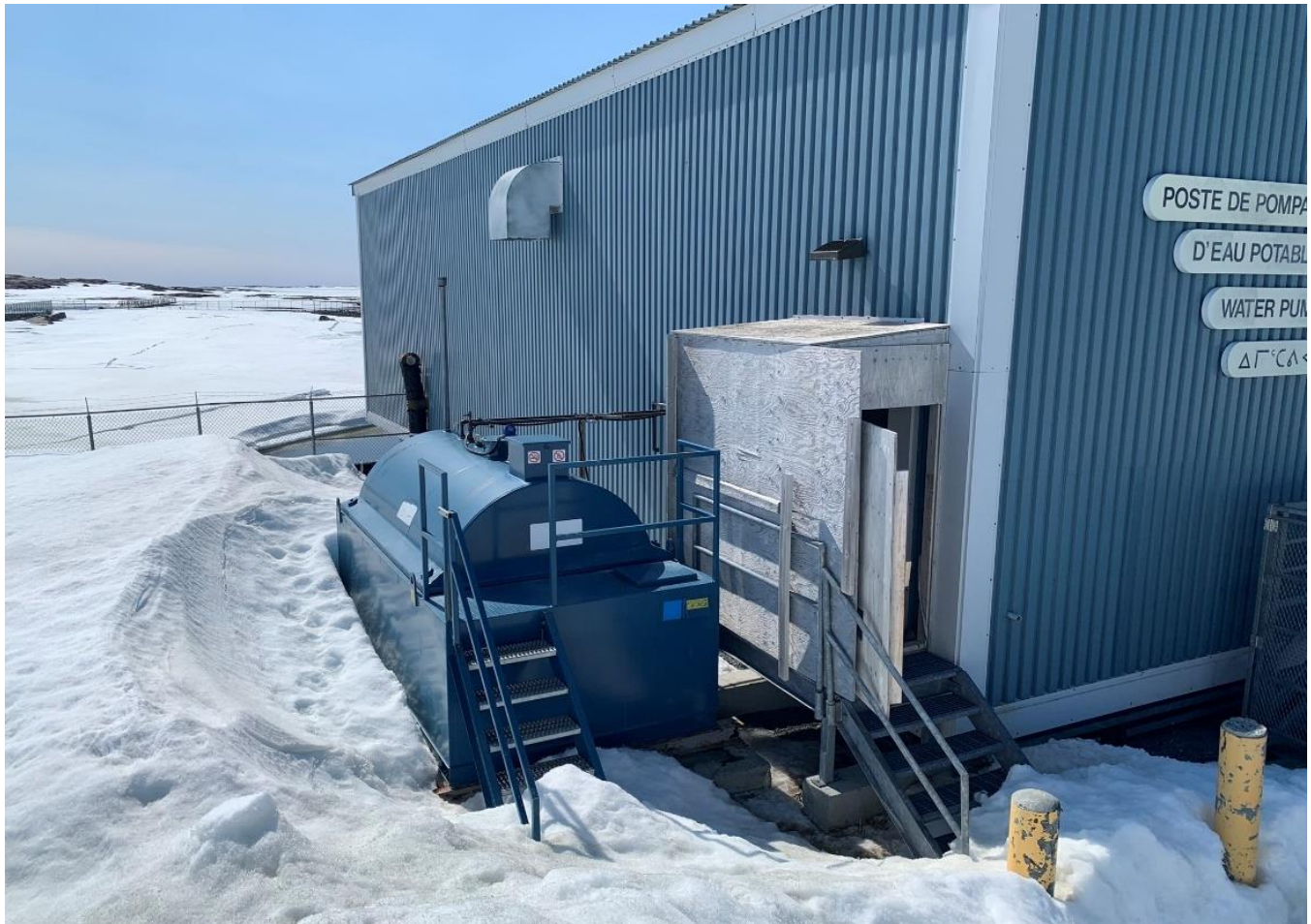
Figure 5. Diesel tank attached to the Akulivik WTP building. Photo taken on May 19, 2024.
