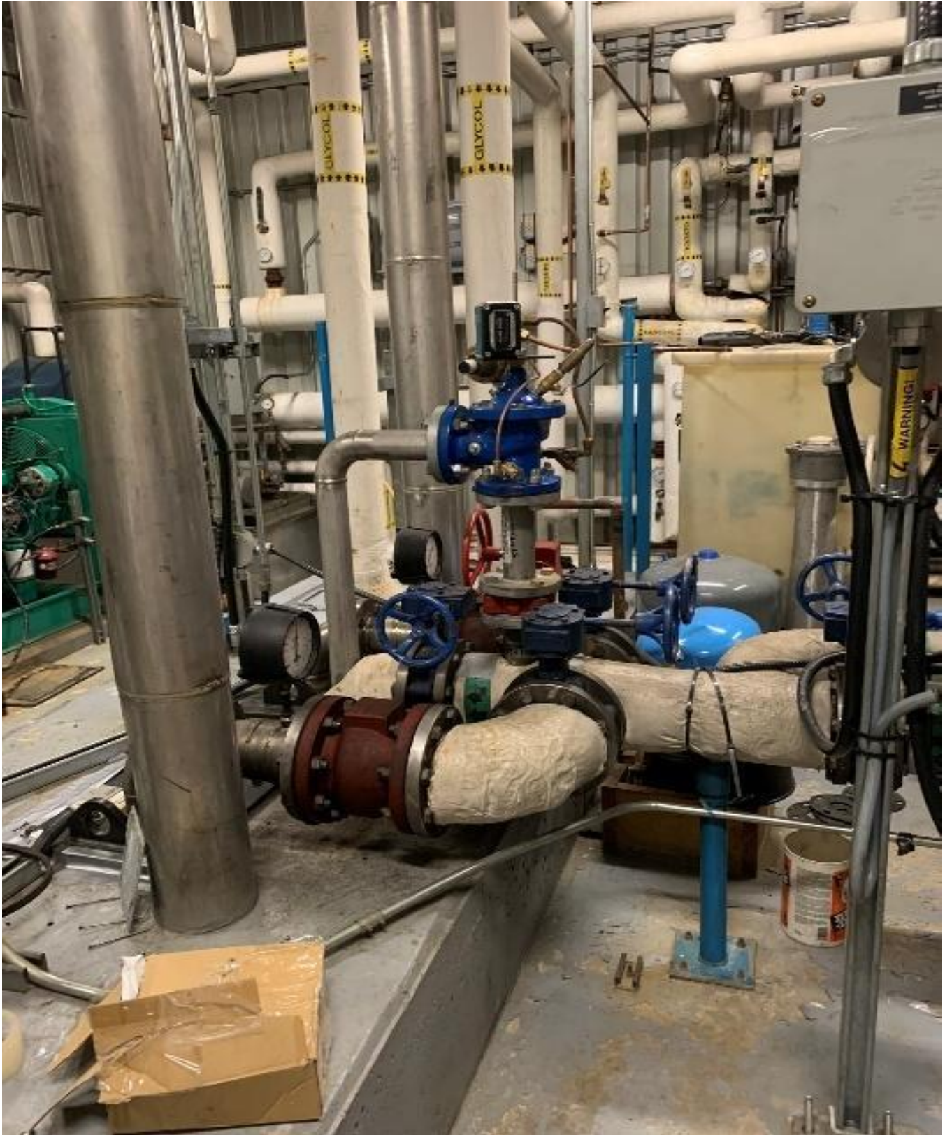
Figure 6. Interior of the pumping station. Photo taken on May 16, 2024
