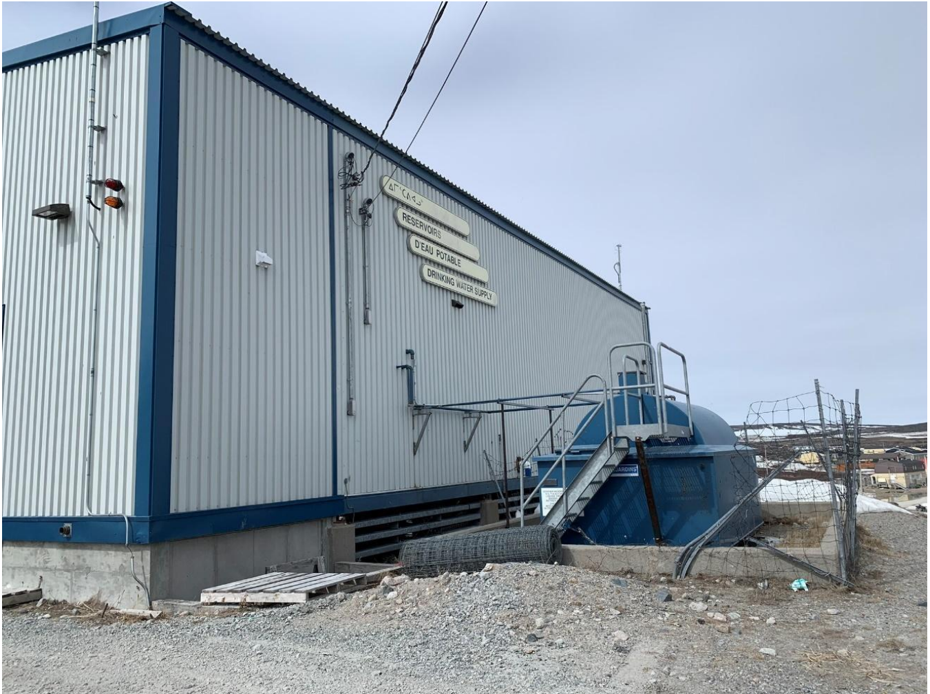
Figure 8. South face of drinking water production building with view of oil tank (photo taken on May 16, 2024)
