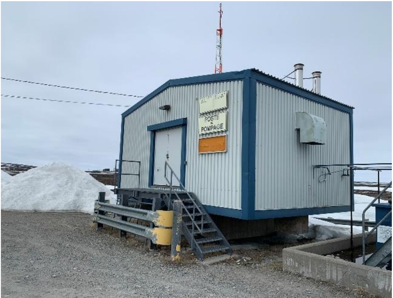
Figure 4. Exterior view of the Inukjuak pumping station. Photo taken on May 16, 2024
