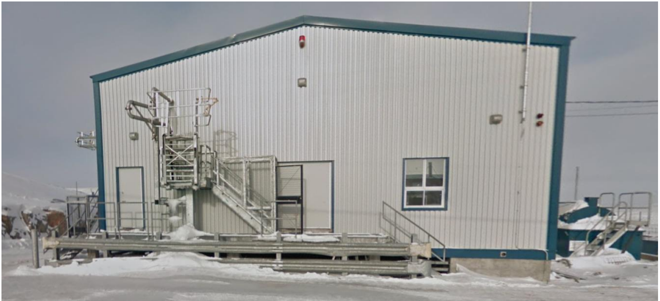
Figure 7. Inukjuak drinking water production facility (Photo: Google Earth)
