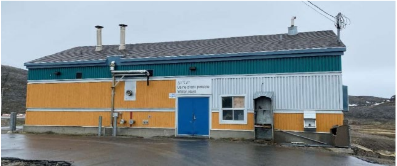
Figure 6. Drinking water treatment plant in the Northern village of Kangiqsujaq [8].
