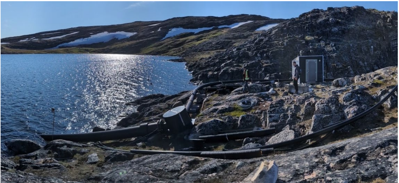
Figure 3 Supply conduit and submersible pump used to withdraw water from Lake Qurlutuup Tasinga
