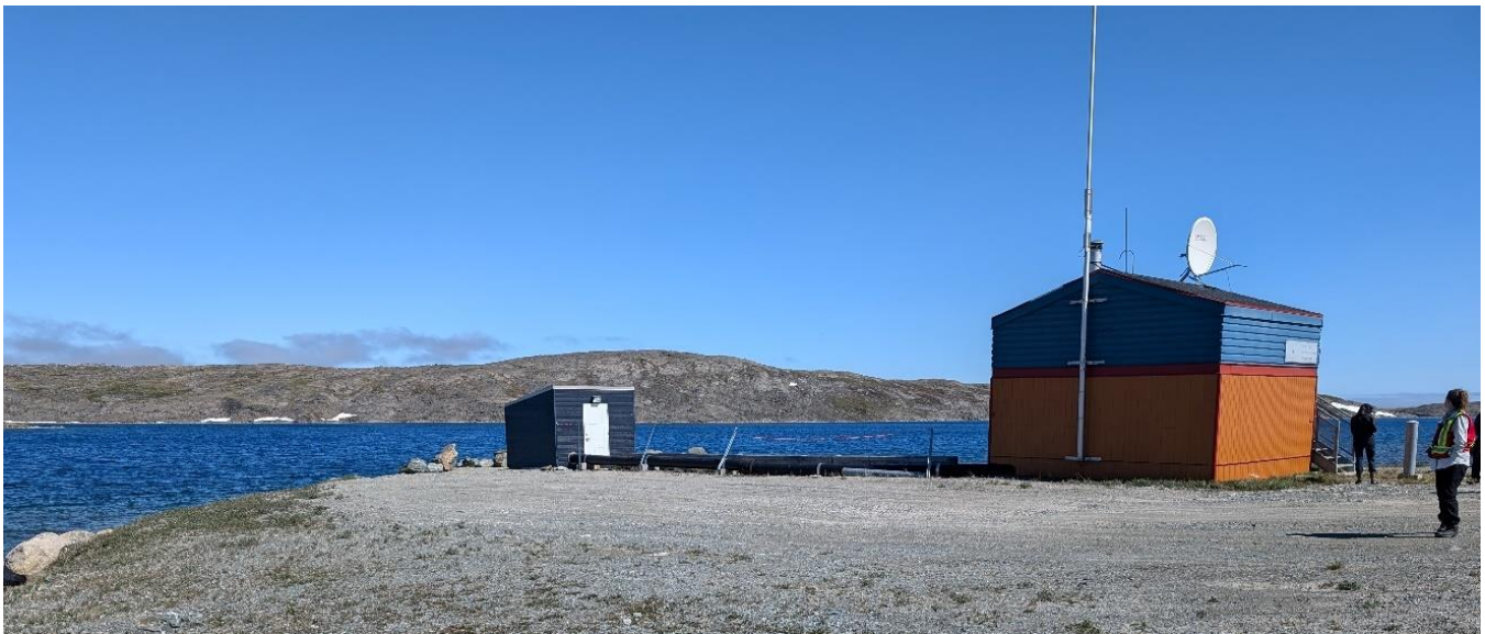
Figure 3. Drinking water withdrawal infrastructure. The navy blue building houses the pumps (Photo taken on July 18, 2024, by Antoine Thibault)
