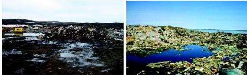
Municipal waste disposal site operators must ensure that surface water does not flow through the waste. Water infiltration in the waste would contribute to the formation of leachate (contaminated water) which can lead to groundwater river and lake contamination. Water falling on and running across the site has the potential to spread disease and contaminate the environment. In addition, storm water runoff can cause erosion.
