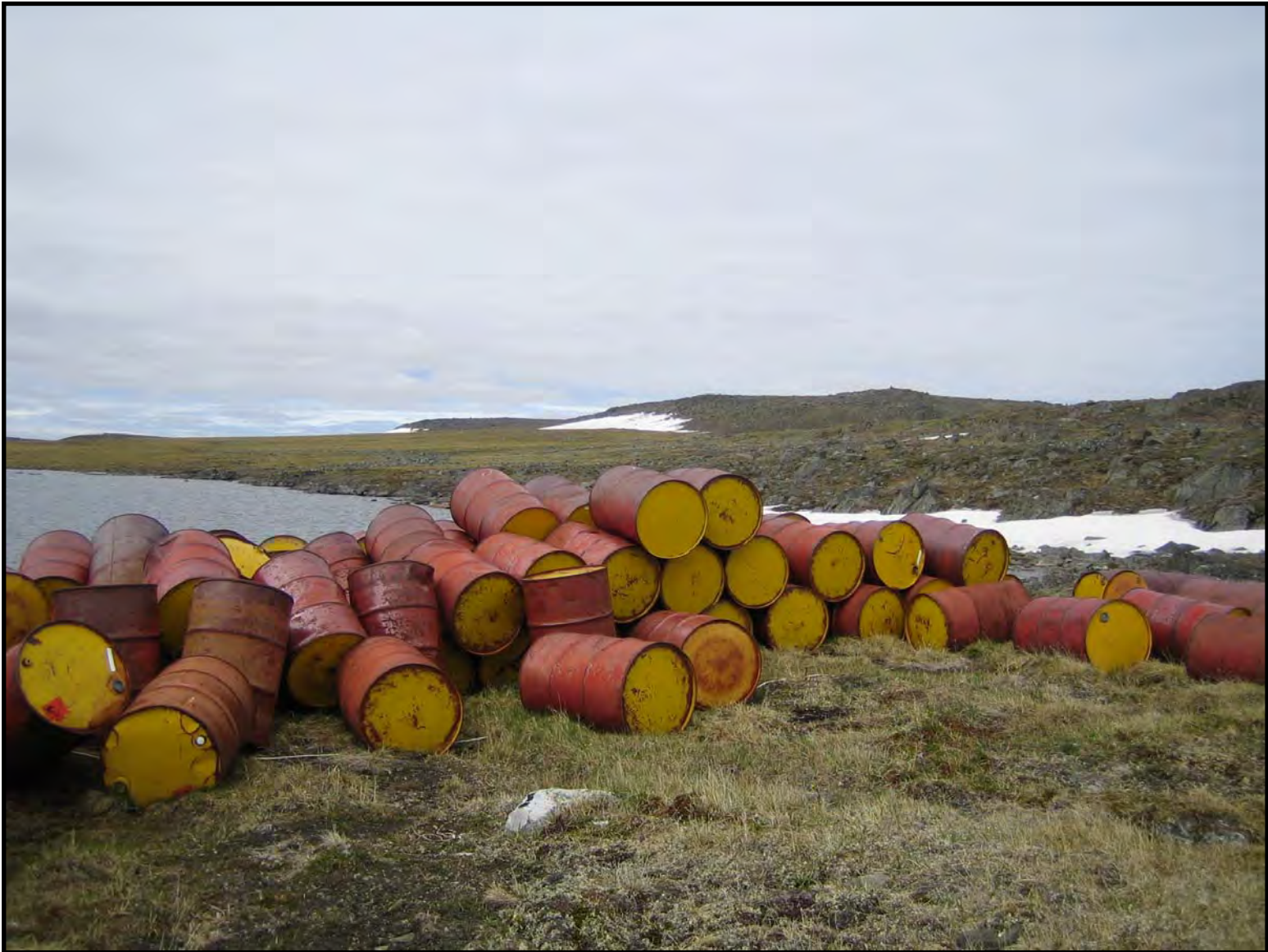
Photo 3. Pile of old fuel drums at the abandoned camp near Lac Dumas, Nunavik, before commencement of AAEC's clean-up effort. A total of 30 drums of fuel were transferred to new drums (6 gas, 24 diesel) and 75 empty drums were brought to Belanger camp in 2005. View looking west, July 7 th , 2005.
