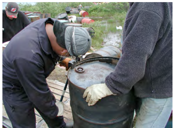
Picture 6. Manual barrel “deheader”.
