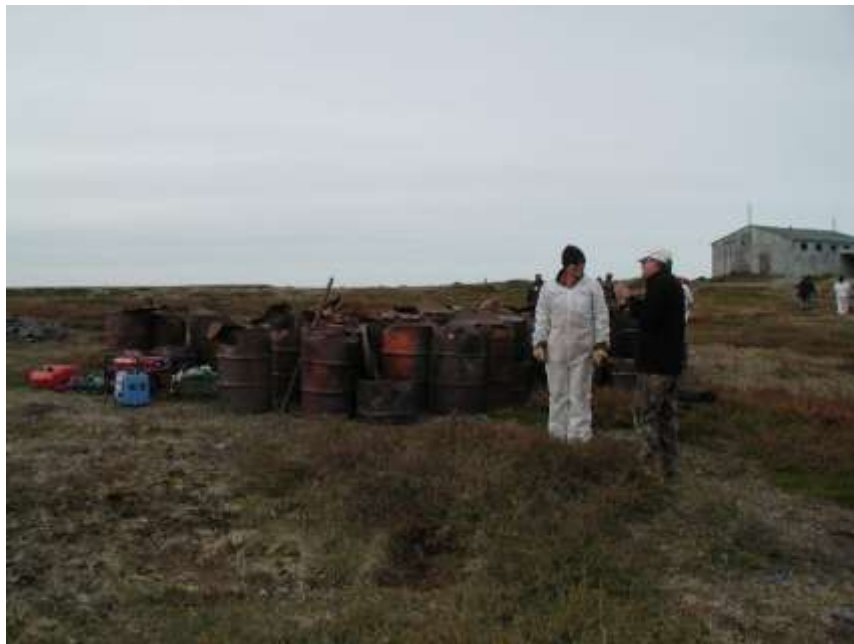
Figure 136: Site PJ-17. Sector shown in Figure 135 during clean-up work. All the barrels were cut up, emptied and removed from the site.
