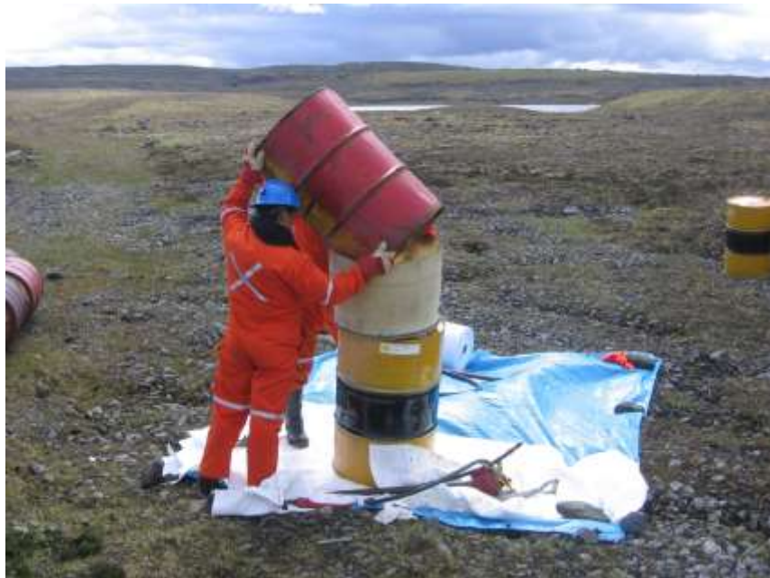
Figure 143: Site SW-34. Residue being transferred to an undamaged barrel using a funnel.
