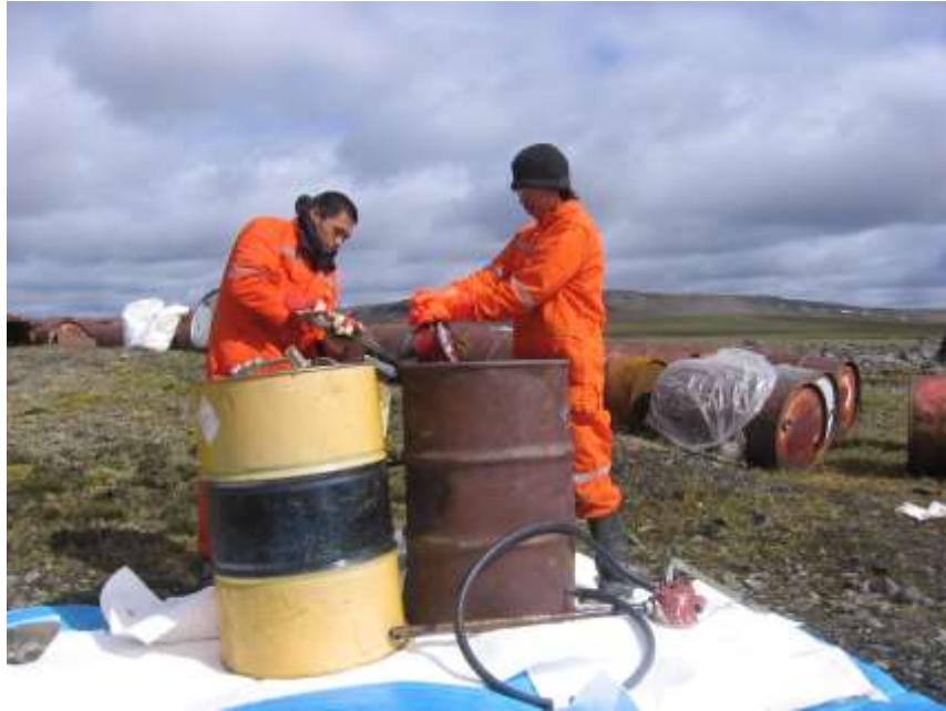
Figure 142: Site SW-34. Residue being transferred to an undamaged barrel using a manual pump.
