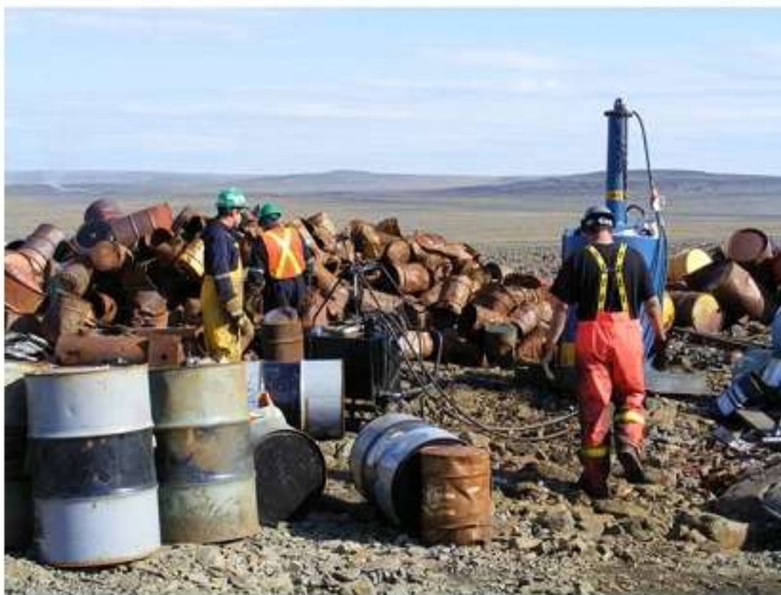
Picture 2 - Crushing of barrels for transportation - K-61
